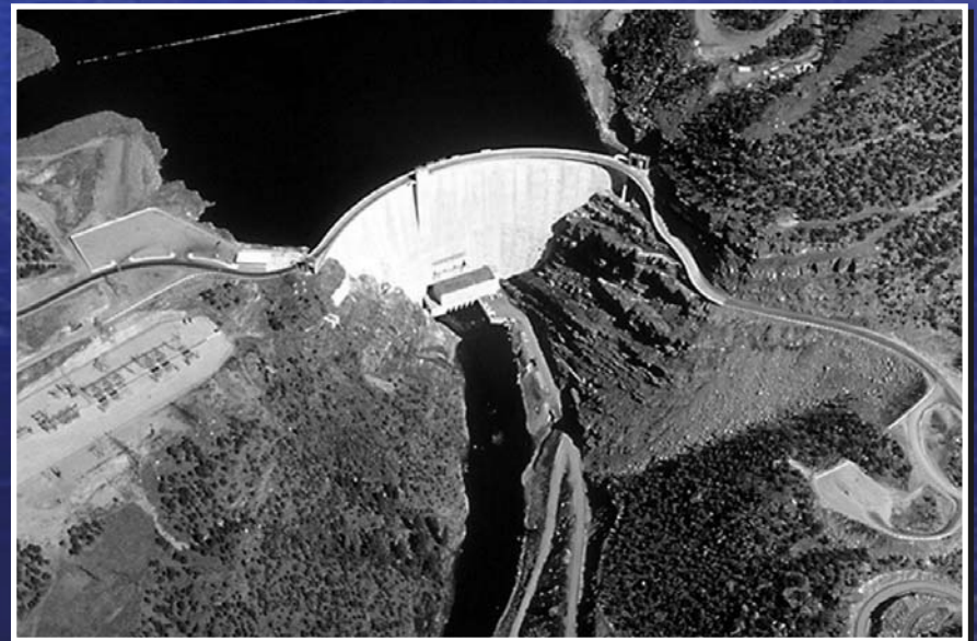
Flaming Gorge Dam On the Green River
