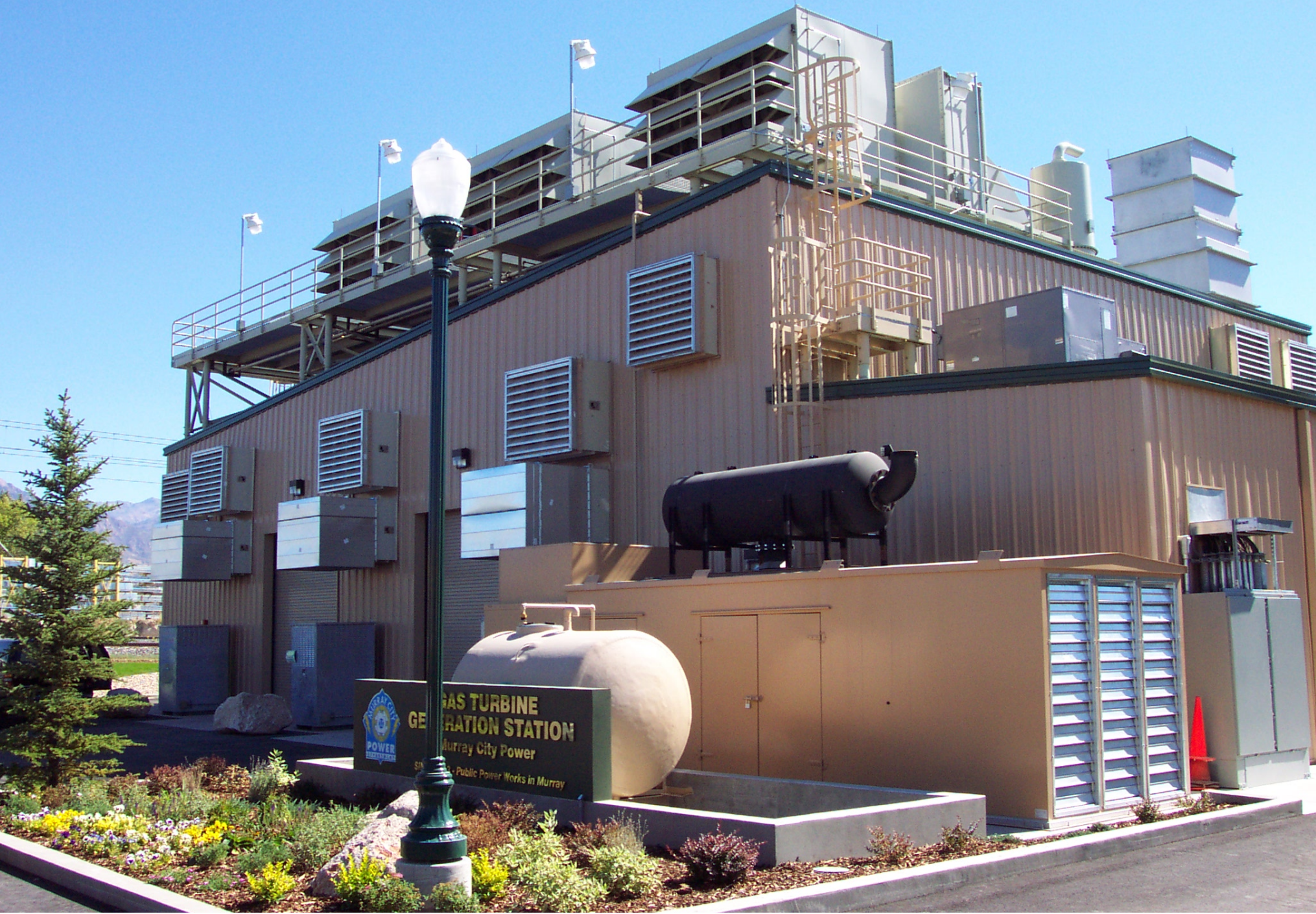
Gas Turbine Generation Station
