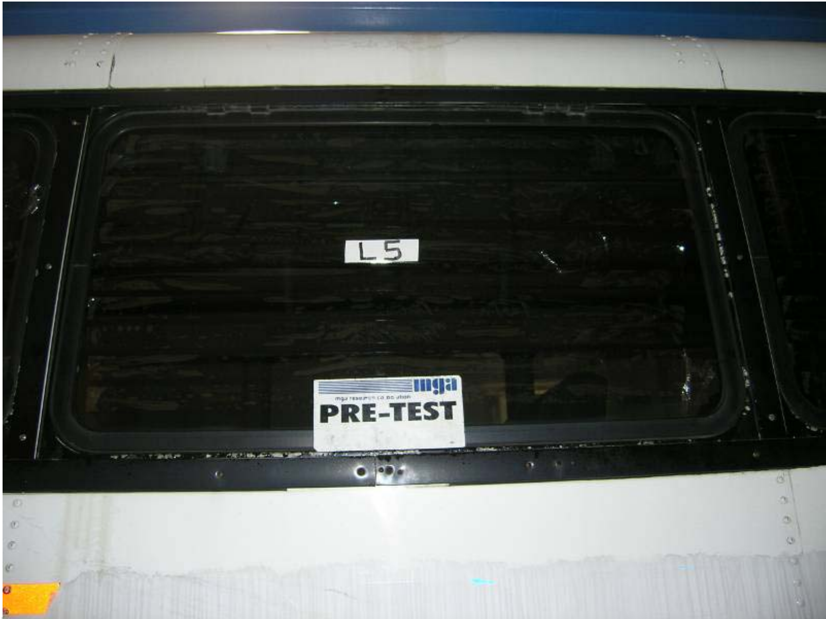
Pre-Test Left Side Window 5 Exterior View
