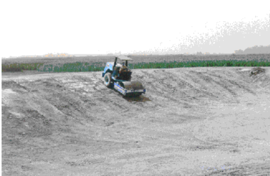
Figure 12. Final Smooth Rolling of FGD..
