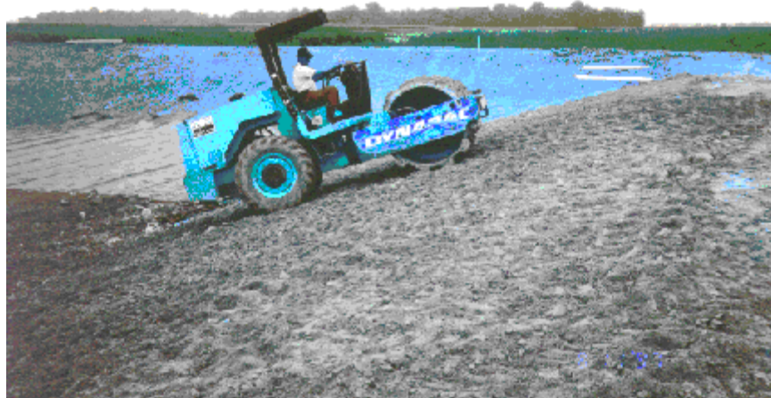
Figure 11. Compacting FGD on a Side Slope.
