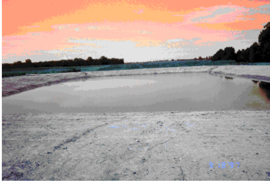
Figure 14. Facility Filled With Water.
