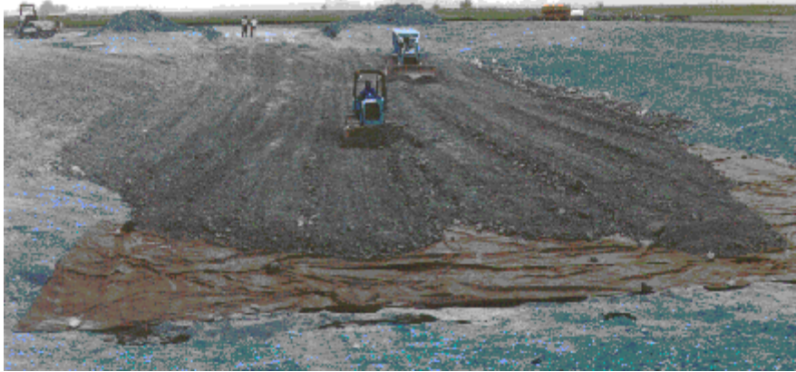
Figure 10. Spreading the FGD.
