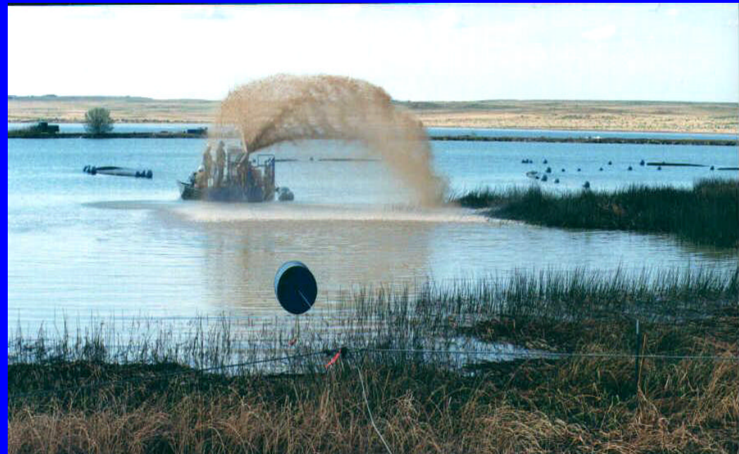
Spraying sand slurry into shallows
