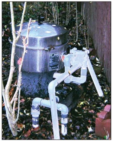
Figure 14.2. Typical Home Pool Equipment System
