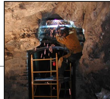
Installing a new cave gate
