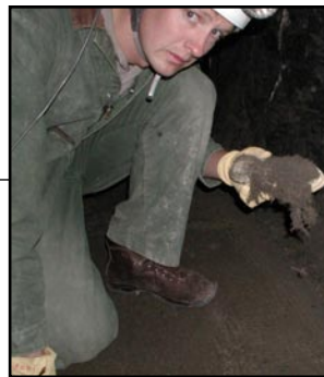
Lint and hair being removed from tunnel
