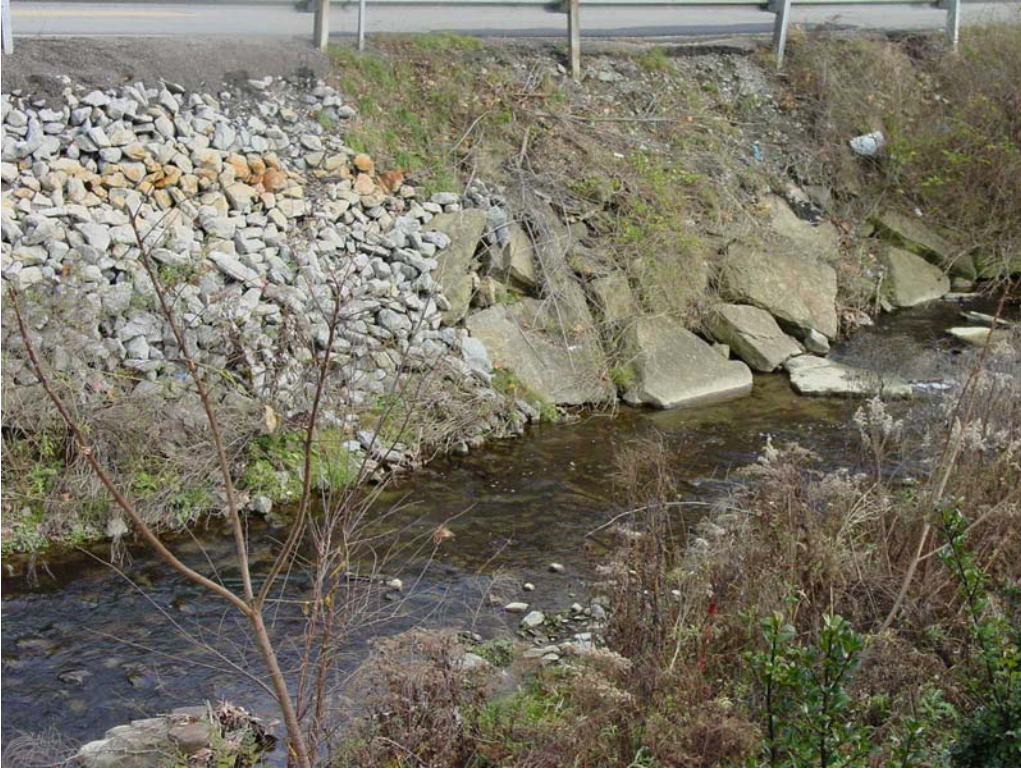
Figure 6 - Typical of the armored banks necessary to convey high water events without causing damage to roads.
