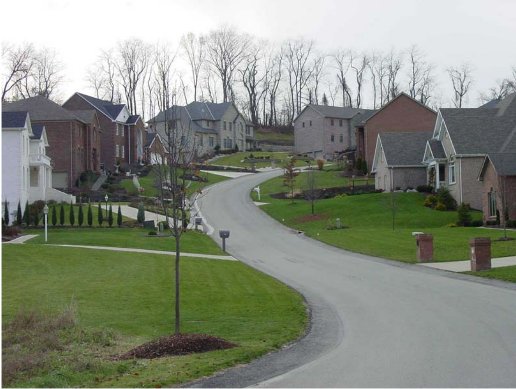
Figure 12 - Example of development on steep slopes with little or no runoff controls or retention.
