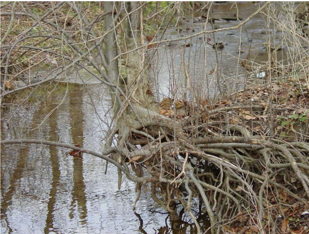
Figure 7 - Increased water velocity and increased bank scour results in the undercutting of trees.
