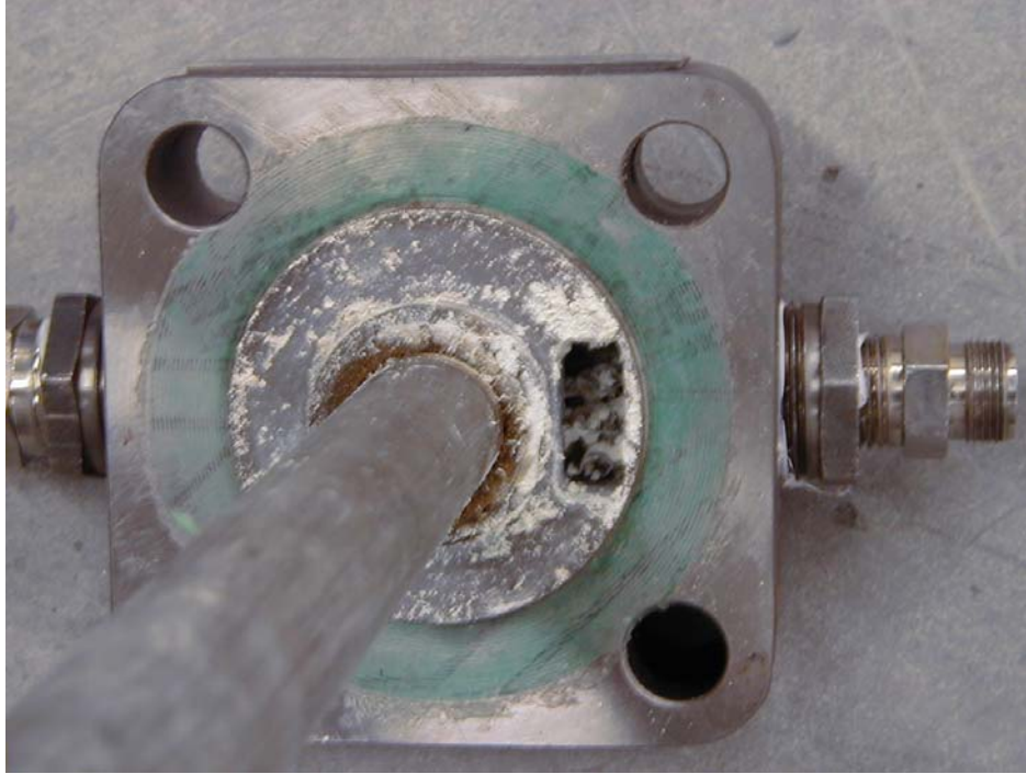
Figure 3.31. Inlet Port of the Nowata Housing that Filled with Packing and Plugged During the First Cycle
