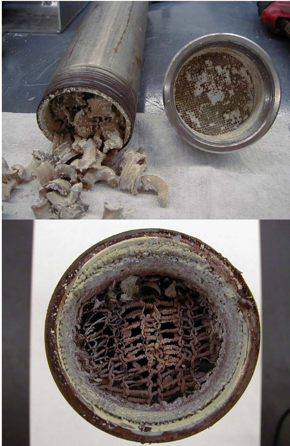
Figure 3.30. Intalox Ceramic Packing (top) and Wire Mesh (bottom) in 2 in. Schedule 40 Stainless Steel Knockout Pot. Condition after three test cycles.
