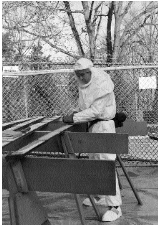
Any mechanical scraping or paint removal with a heat gun will require the operator to wear, at a minimum, a half-face respirator fitted with High Efficiency Particulate Air (HEPA) cartridge filters. This worker is fully suited and wearing a full-face respirator because extensive paint removal is under way.
