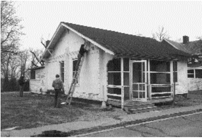
A risk assessment of the property is recommended when lead-based paint is present. The paint's location and condition should be recorded and a list of priority risk areas should be identified. Deteriorated paint and friction surfaces on windows and doors should be treated first.
