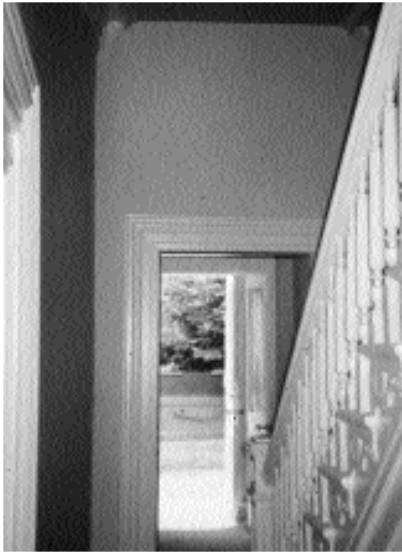
Some residential properties scheduled for full hazard abatement may require a greater level of paint removal or encapsulation than non-residential properties. In this instance, loose deteriorated paint was wet sanded and then the trimwork was painted with several thin layers of a special encapsulant paint coating.
