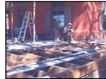
Front Porch of TRH under repair
