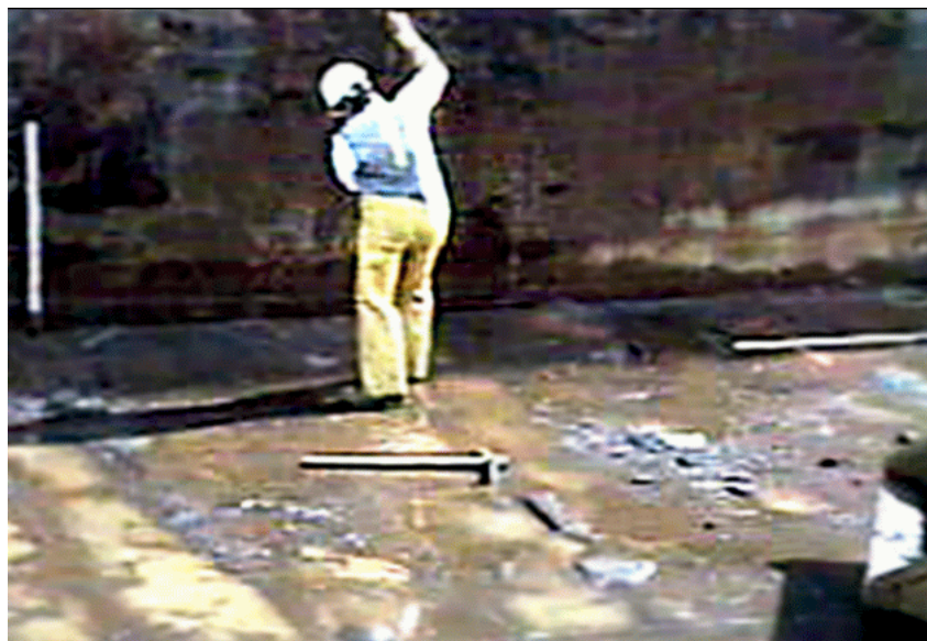
Figure 6. Employee using “spud” bar to break up asphalt on barge. Manual application and reaction forces to and from the spud bar may cause musculoskeletal disorders, especially when combined with high repetition and force.
