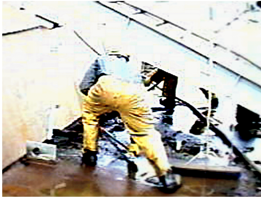
Figure 6. Employee using “spud” bar to break up asphalt on barge. Manual application and reaction forces to and from the spud bar may cause musculoskeletal disorders, especially when combined with high repetition and force.
