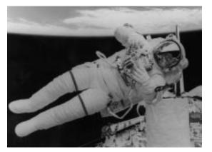
During the first untethered space walk in 10 years, Mission Specialist Mark Lee tests the new Simplified Aid for Extravehicular Rescue (SAFER) system. The 28th space walk of the Shuttle program took place on Mission STS-64 in September 1994
