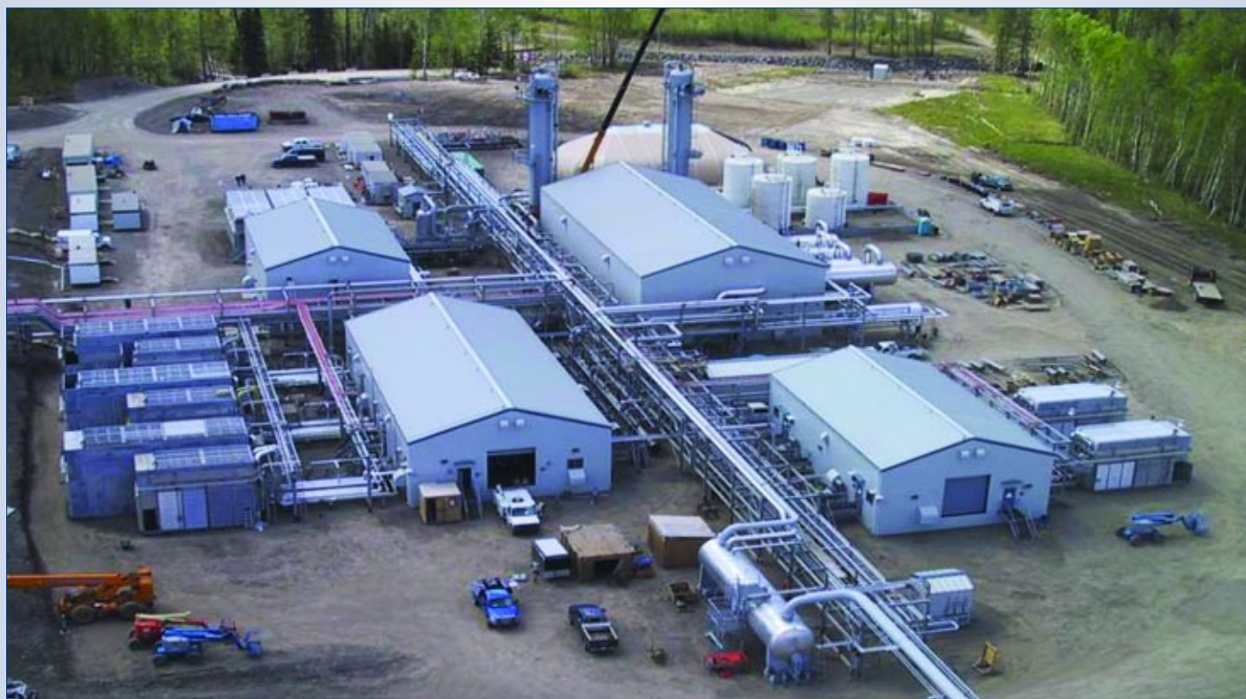
Figure 3: The Kwoen plant was completed in August 2002.
