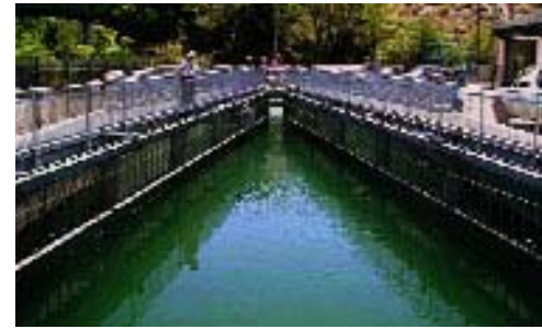
A new fish screen and two fish ladders on the Sacramento River will save millions of tiny Chinook salmon fry and allow hundreds of adult fish to reach upstream spawning habitat. PHOTO: SOUTHWEST REGIONAL OFFICE
