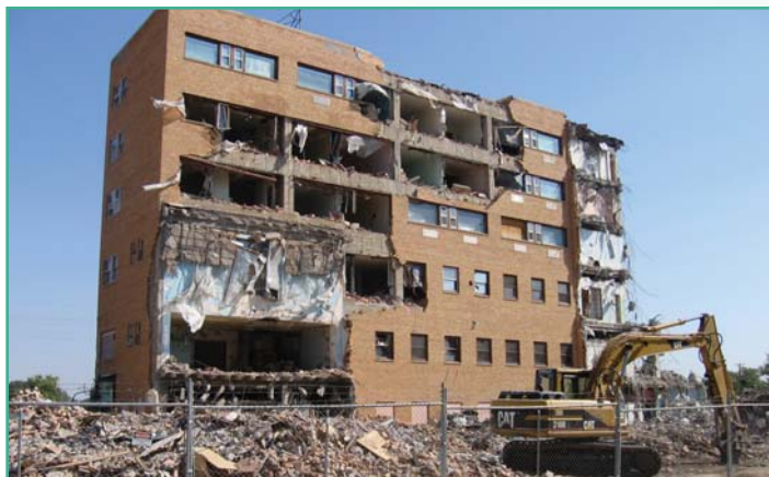
The six-story building during demolition.
