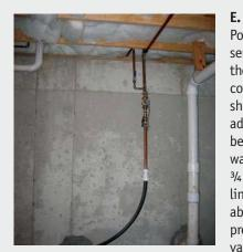
Polyethylene water service pipe entering the home through the concrete basement wall shown. White plastic adapter shown between polyethylene water service pipe and <sup>3</sup>/<sub>4</sub> inch copper water line. A short distance above the adapter is a pressure reducing valve. To the right of
