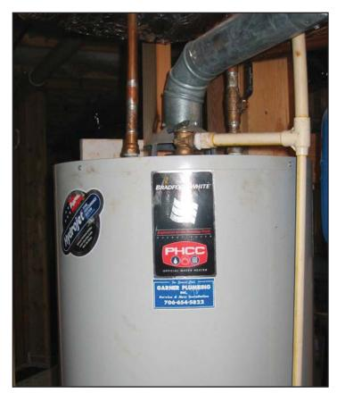
Figure 9.4. Temperature-Pressure Valve
