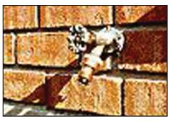
Figure 9.17. Hose Bib With Vacuum Breaker
