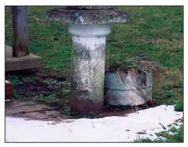
Figure 8.9. Drilled Well
