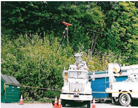
Figure 2-1. Work area showing the pole in the brush
