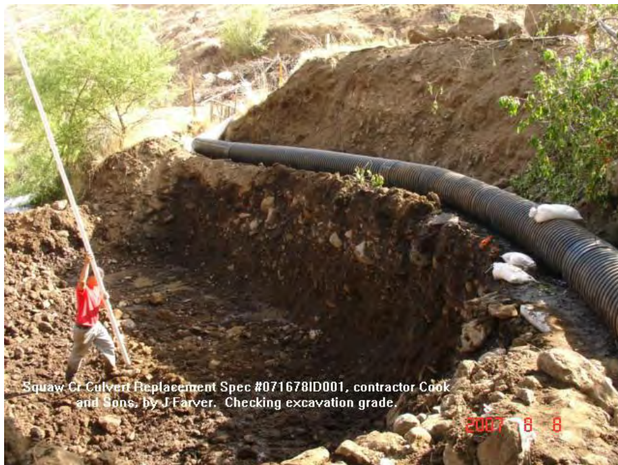
Photograph No. 6. Checking excavation grade. Photo by J. Farver.
