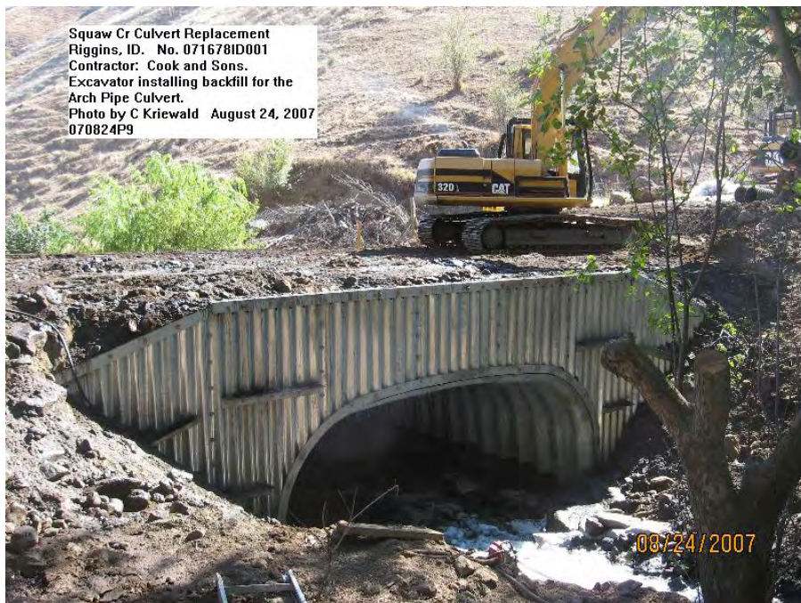
Photograph No. 10. Bottomless arch culvert with wingwalls installed. Photo by C. Kriewald.
