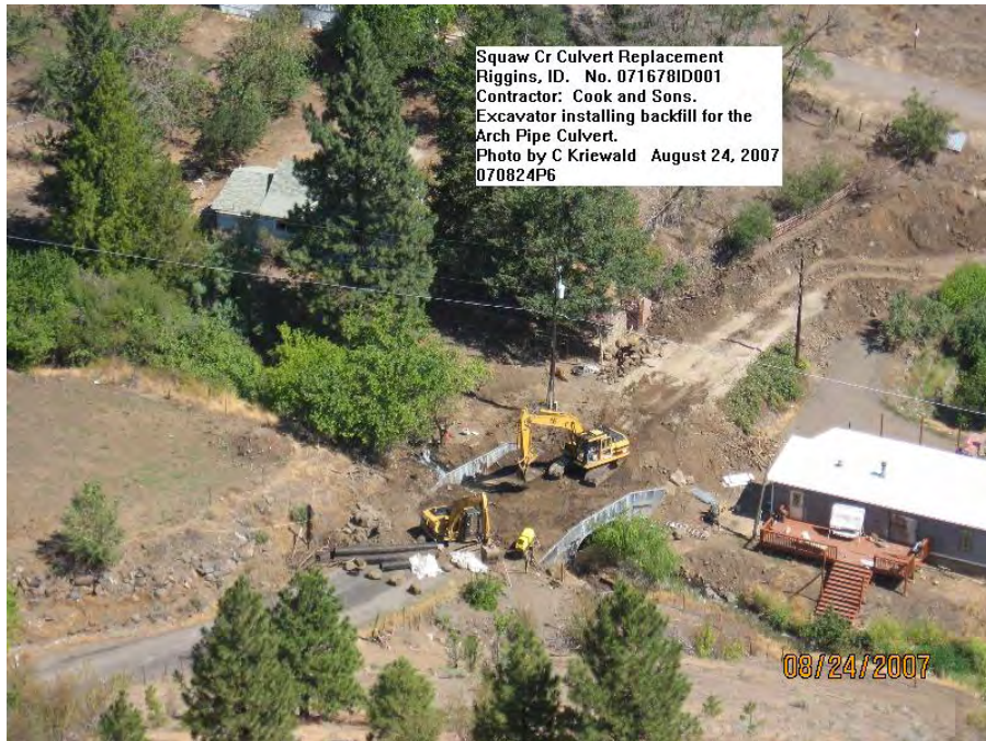
Photograph No. 9. Excavator installing backfill for arch pipe culvert. Photo by C. Kriewald.
