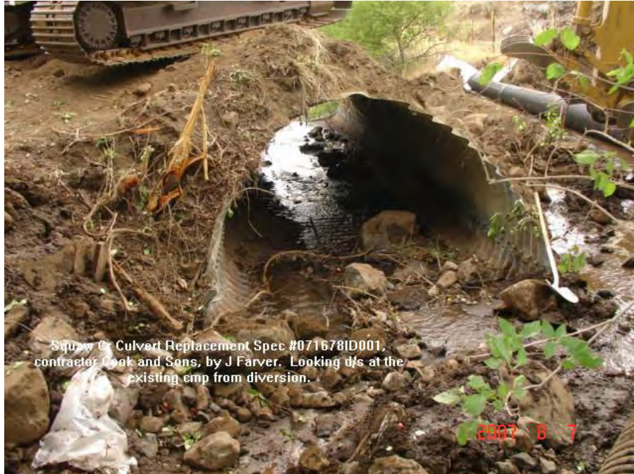
Photograph No. 5. Looking downstream at the existing corrugated metal pipe. Photo by J. Farver.
