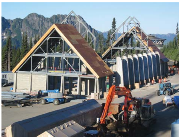
Construction of the new Paradise Visitor Center.
