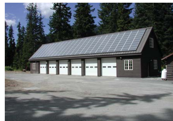
Solar Energy System at White River
