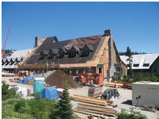
Rehabilitation of the historic Paradise Inn.
