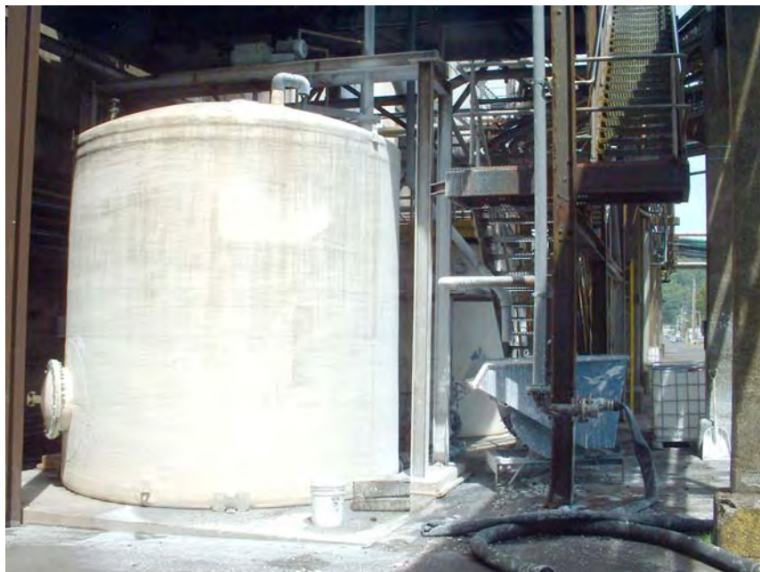
Figure I-3.15-6. Product storage tank and reject dumpster for the product screen.
