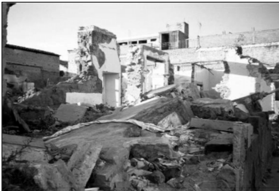
Many of the buildings in downtown Tegucigalpa, Honduras were destroyed by Hurricane Mitch. A Commerce team went to the Central American city to help with the rebuilding.
