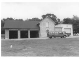
ing contains three garage bays, and the roof is asphalt shingles. An addition with a metal roof, containing a garage service area, was constructed on the right wing in the 1970's.
