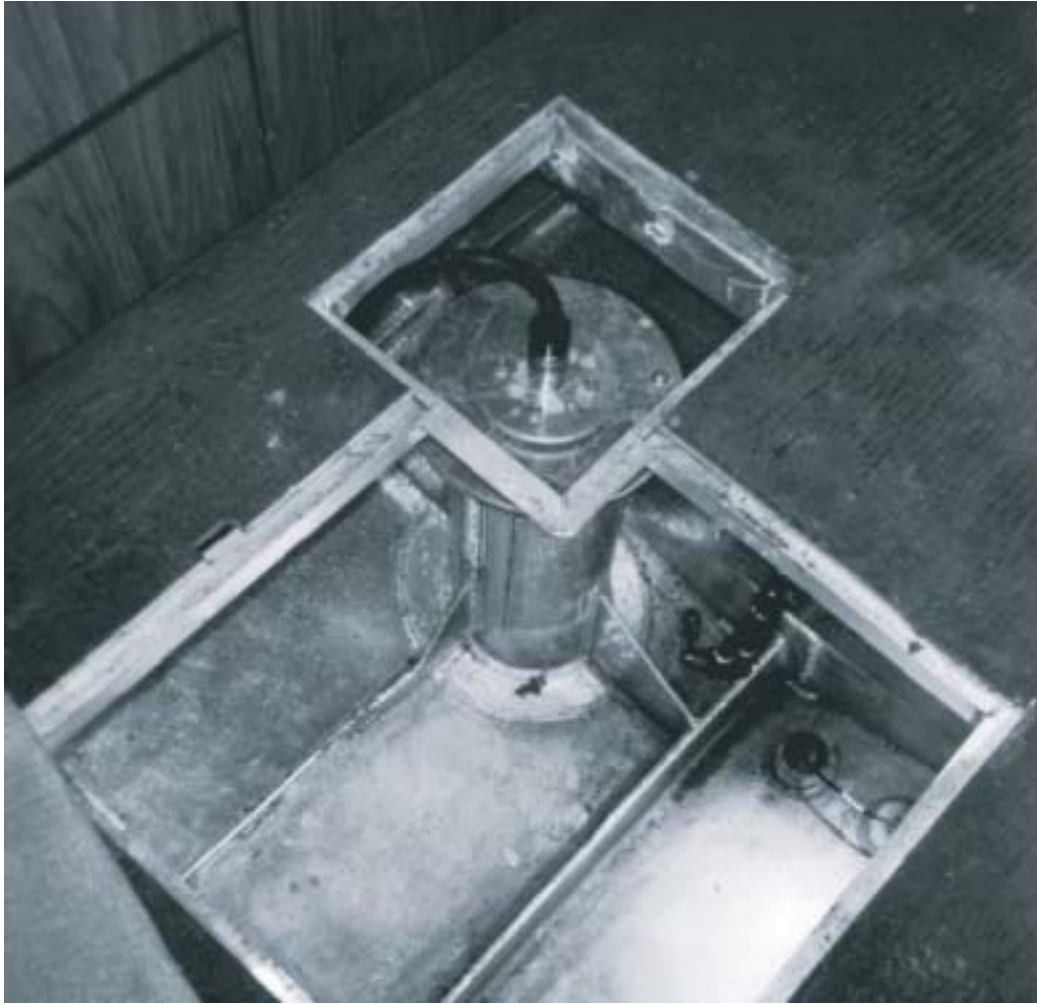
Figure 4.16. Sea-chest mount for a narrow-band acoustic Doppler current profiler.
