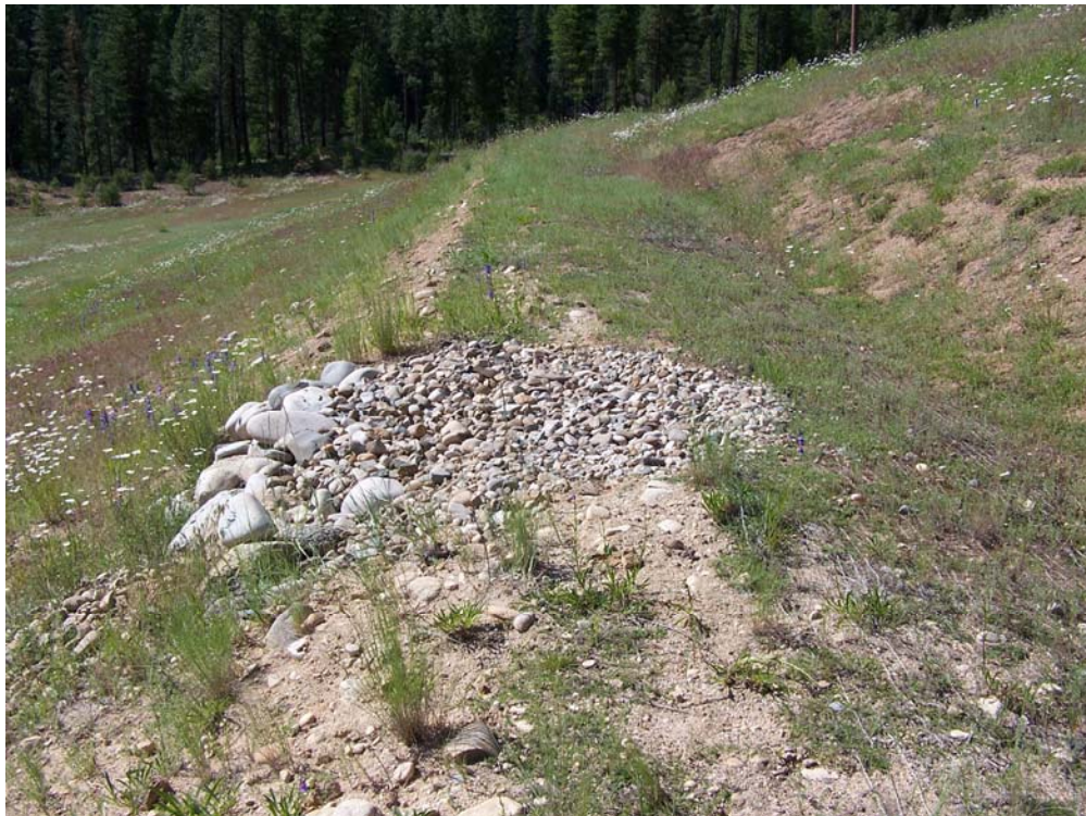
Photo 2. Riprap repair of the downslope portion of middle interceptor bench.
