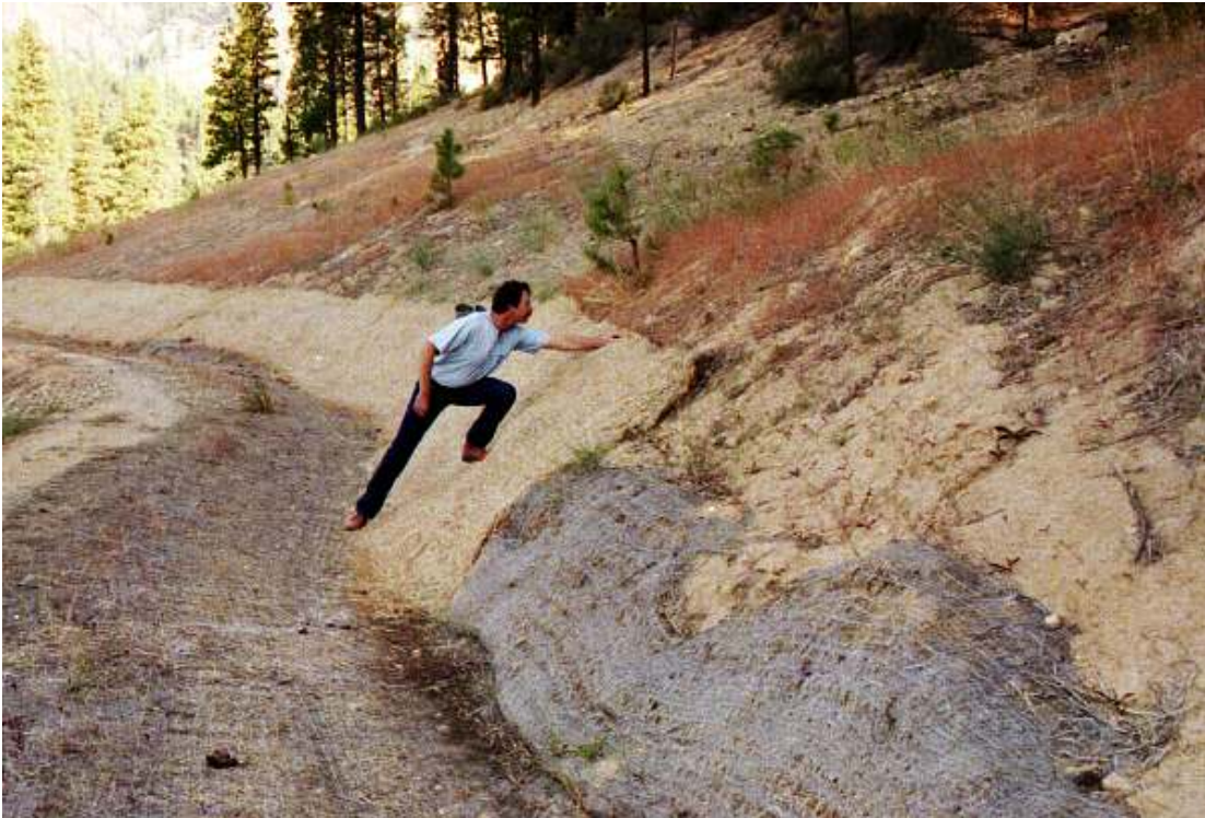
Photo 1. Inspector checking erosion control fabric within the top interceptor bench.
