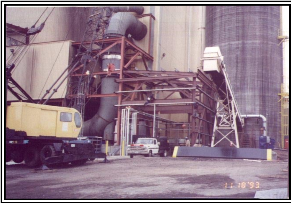
Figure 5.4: Drive-in Sump Under Construction.
