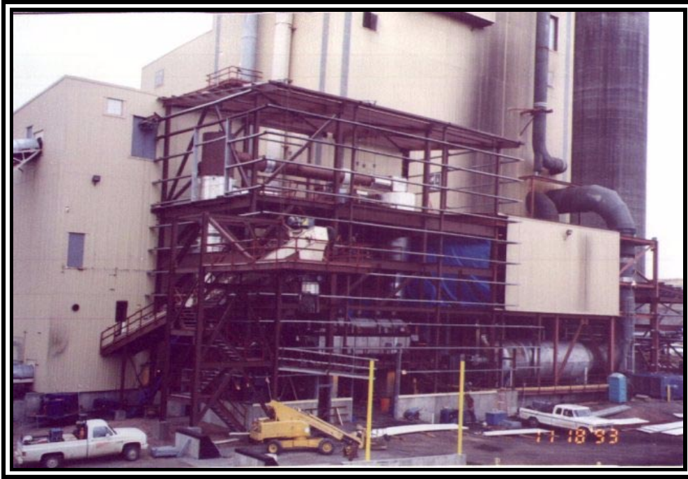
4.5b: PDF Deactivation System Under Construction.
