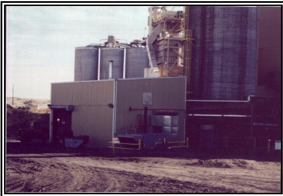
Figure 5.8b: Process Water Fines Removal Building.
