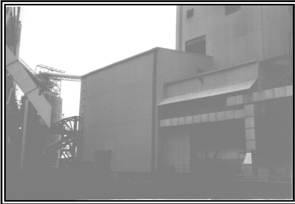
4.5c: PDF Deactivation Building Completed.
