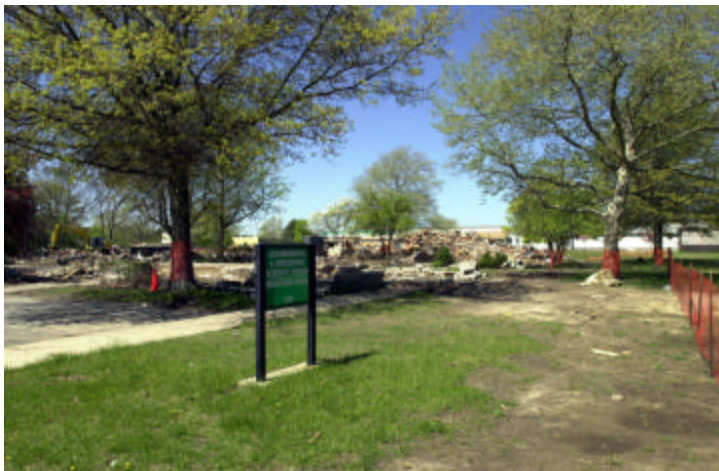
Removal Nears Completion
