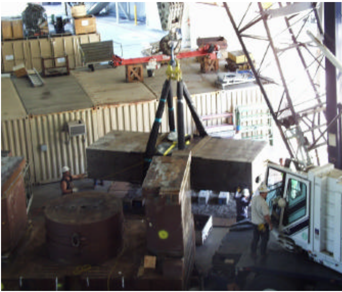
Removal of 106 ton HISS Magnet top piece at LBNL Bevatron
