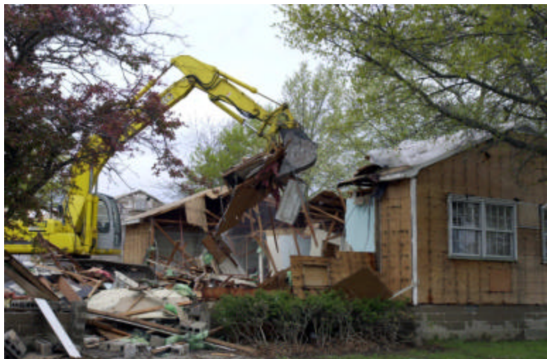
Demolition of Building 318 at BNL
