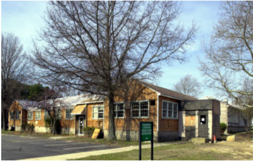
Building 318 at Brookhaven National Laboratory prior to demolition. This 24,708 square foot building was constructed of wood in 1941 and provided office space for the Oceanographic and Atmospheric Sciences Division. It was 61 years old.
