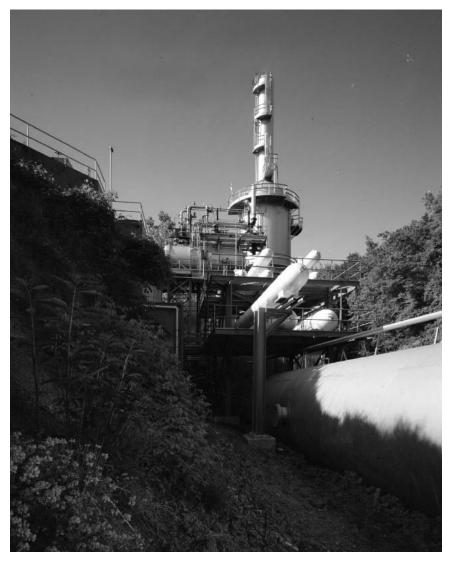
The RETF after the \$1 million modification to create the new altitude facility (Stand B), 1985. This modification made the RETF even more versatile, allowing engineers to rapidly switch instrumentation and control from one test stand to the other. NASA C-85-4093
