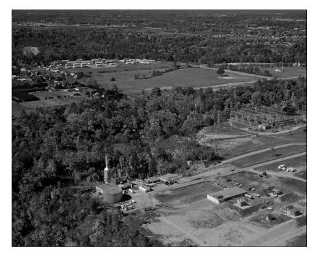
Aerial view of the RETF in 1963. The old rocket engine test cells can be seen (lower right), protected by earthen mounds. The woods separated the RETF from residential areas of Brook Park to the south. NASA C-66584.
