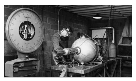
Preparing jet assisted take-off units, called JATOs, for testing in one of the four rocket test cells built during World War II at the Aircraft Engine Research Laboratory in Cleveland, Ohio.
