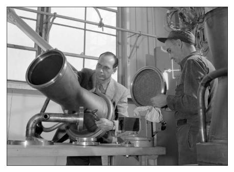
Engineer Walter Russell (left) from the Fabrication Division inspects a regenerativelycooled thrust chamber for a 20,000-pound-thrust rocket engine while a technician cleans the face plate of an injector in the shop of Building 100, 15 Dec. 1958. NASA C-49343.
