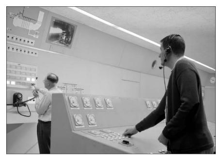
Operations engineers in the control room, located in Building 100, monitor early rocket tests, 1957. Video cameras in the test cell transmitted images during rocket firing. Instruments recorded pressures and other data that was later analyzed by the research engineers in charge of a particular test program. NASA C-45021.
