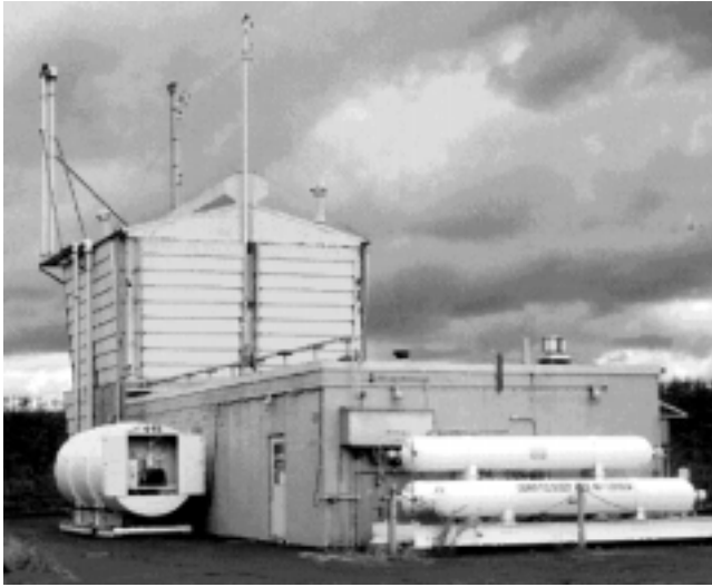
Figure 1.—Supplemental multilayer insulation research facility.
