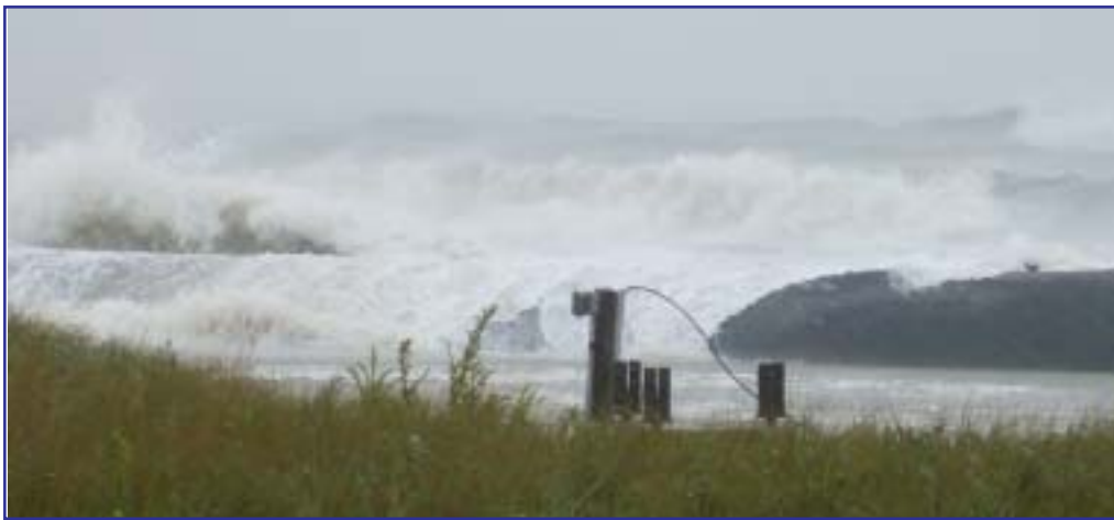
The heavy rain, winds and high tides from last week's N'easter sent the surf crashing over the geo tubes and bulkhead on Wallops I sland.
