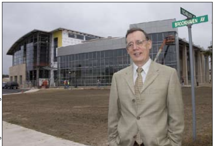
Emilio Mendez in front of the construction site of Brookhaven's Center for Functional Nanomaterials
