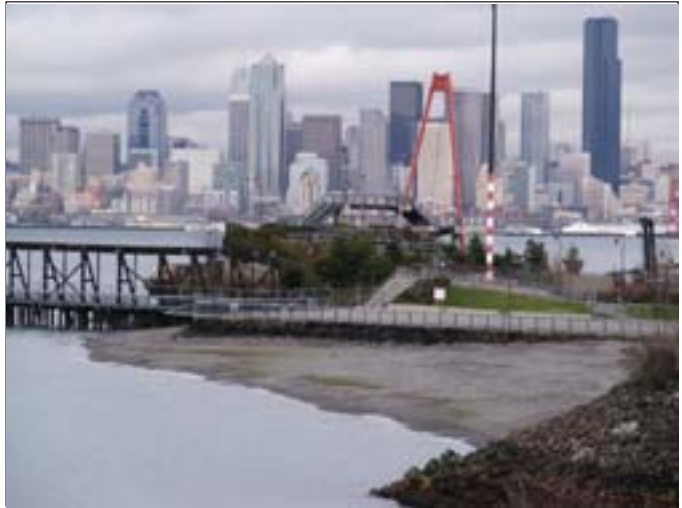
The cap created new beach next to the public park. (Photo courtesy of U.S. Army Corps of Engineers)
