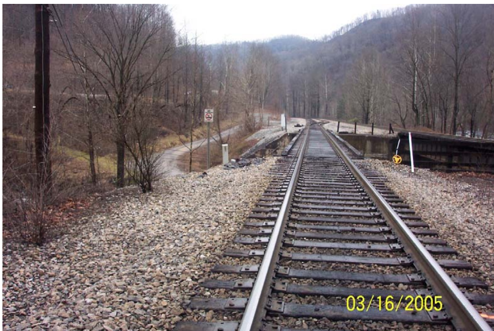
Photo 4. Main #1 looking to the west from west of tunnel (Main #2 on right)
