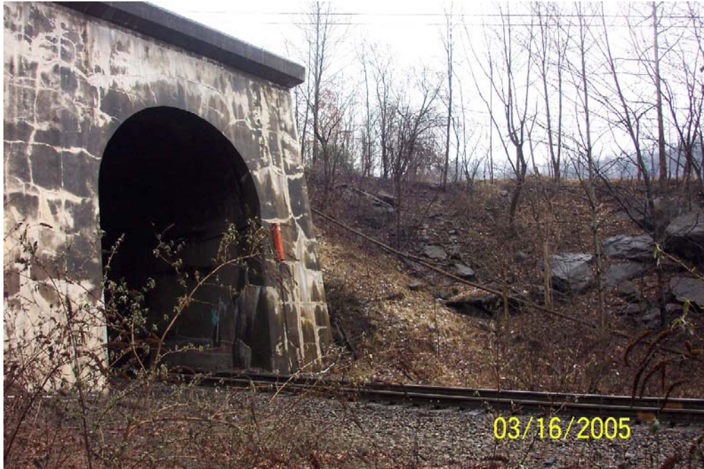
Photo 3. Main #1 west portal
