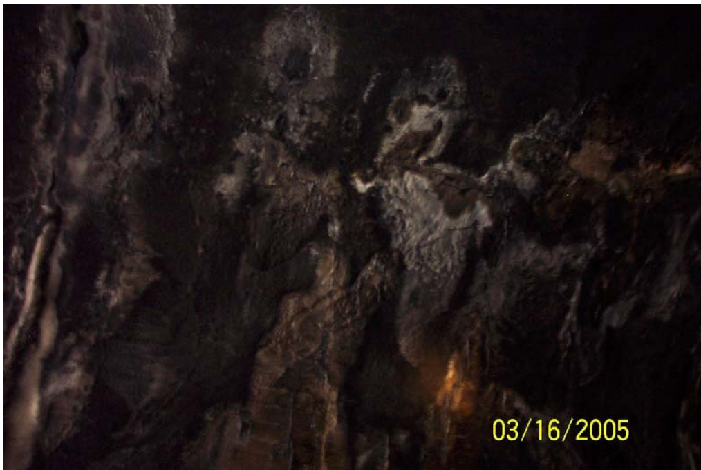
Photo 6. Significant spalling, efflorescence, and leaking from crown, about 70' from west portal of Main #1.
