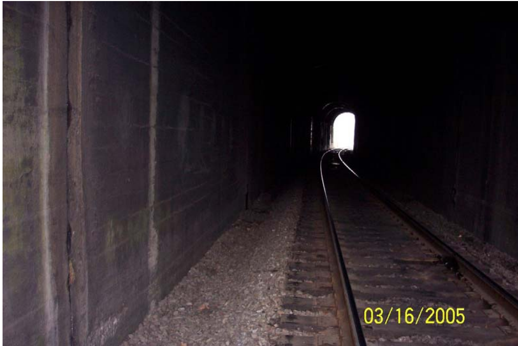
Photo 5. Main #1, looking west from inside east portal
