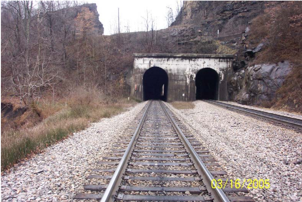
Photo 1. Main #1 east portal (Main #2 on right)
