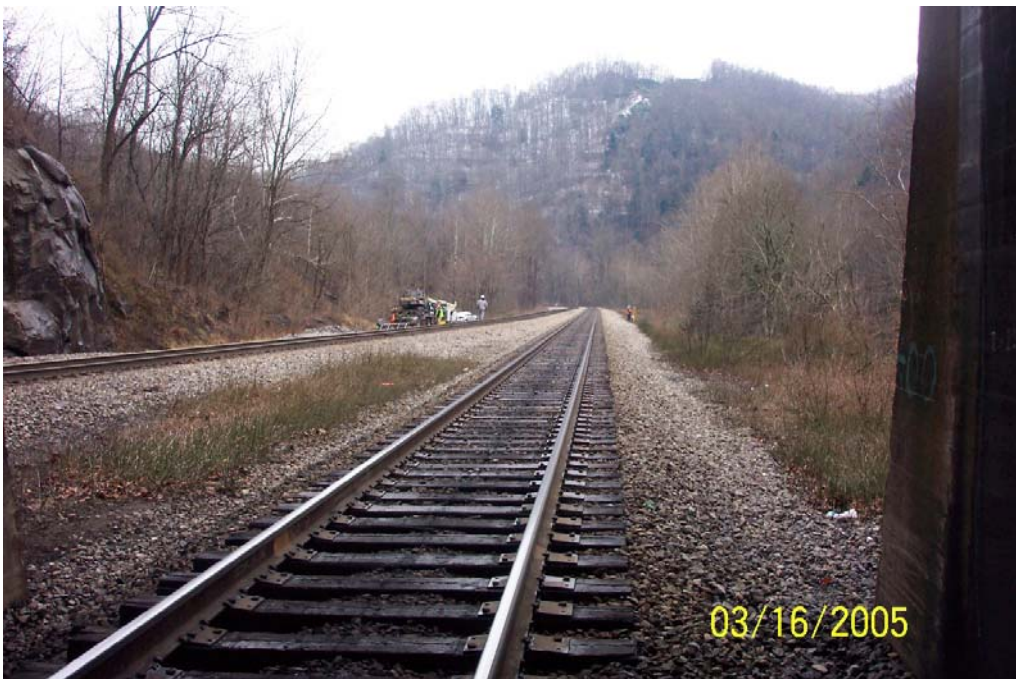
Photo 2. Looking to the east on Main #1 from the east portal (Main #2 on left)
