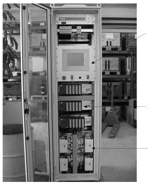
PLC for low-level safety/interlocks -axis monitoring to avoid excessive taper and motor failures -interlocks (motor end stage failure, brake air pressure failure, etc.) -local operation -binary input/output to IOC
