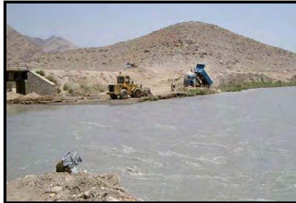
Constructing a spike to divert water-flow away from protection wall
