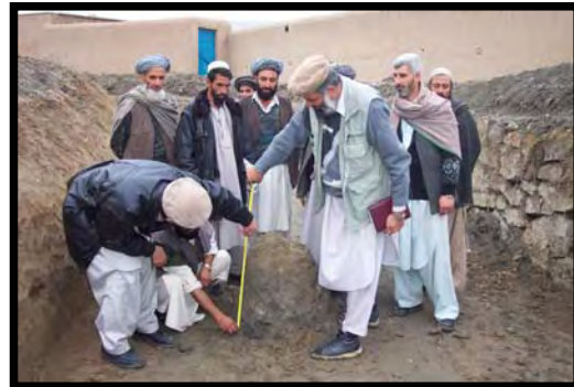
Engineers measure a stump indicating the level of silt that has been removed from Bala Doori
