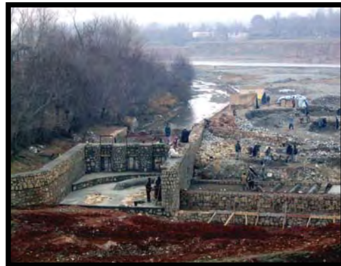
6 January 2004 – during intake construction
