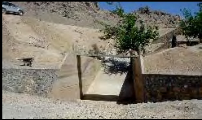
The repaired chute and rebuilt wing-walls
