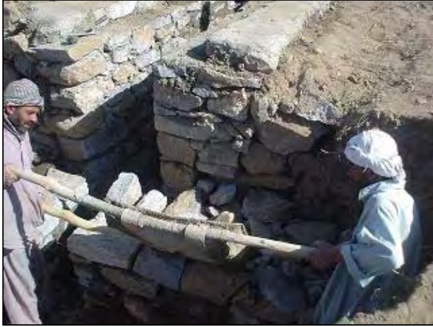
LEFT – Building a water outlet on the Nahri-Charikar Canal
