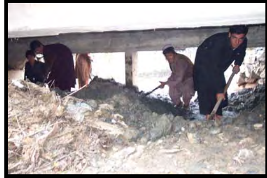
Digging out the Bala Doori as it passes under a road
