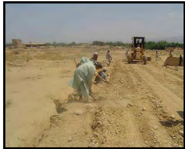
Rebuilding the Darqad farm to market road system.
