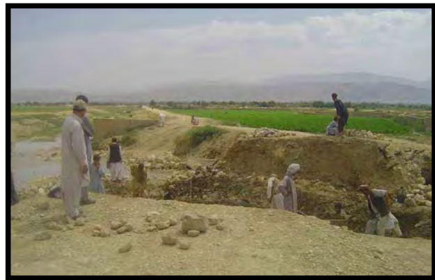
Workers construct a bridge on the Darqad road (above).
