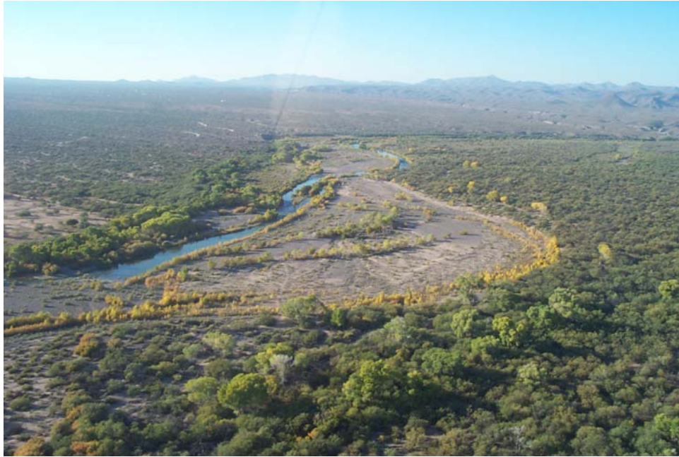
Plate 3. View upstream of Site 3 in the upper part of the picture. The right valley wall is composed of old alluvial and fan sediments, and the left valley wall is comprised of the older and younger Lehi terraces. The larger cottonwoods are growing on the Lehi terraces. Younger riparian vegetation is located on the margins of the active and chute channels.
