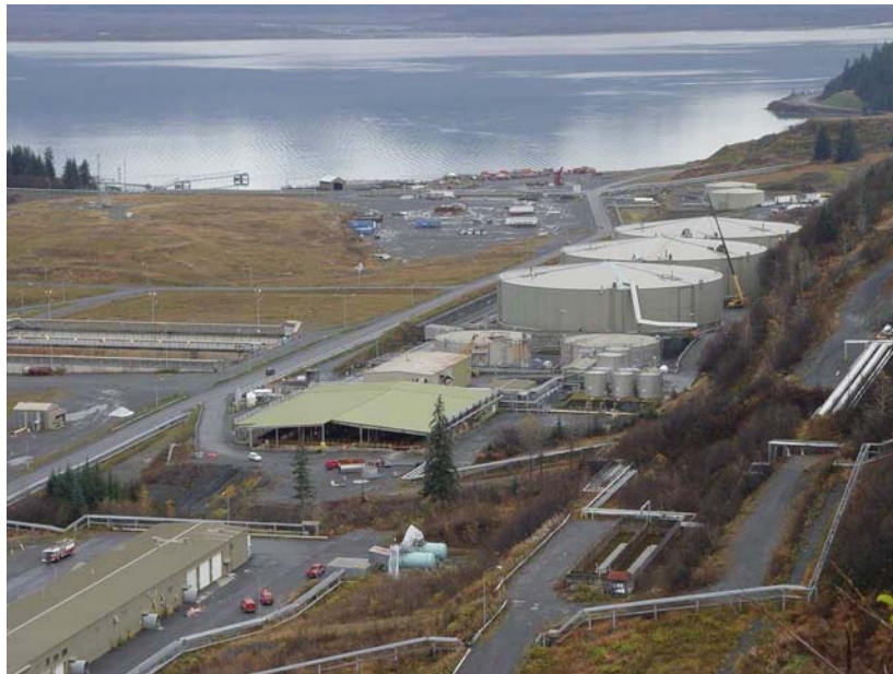
Overview of Ballast Water Treatment Facility (Courtesy Alyeska Pipeline Service Company)
