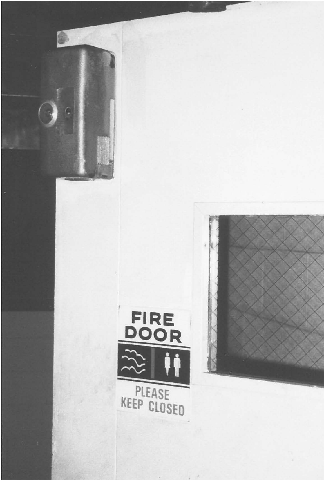
12. Typical door alarm on each stairwell door.
