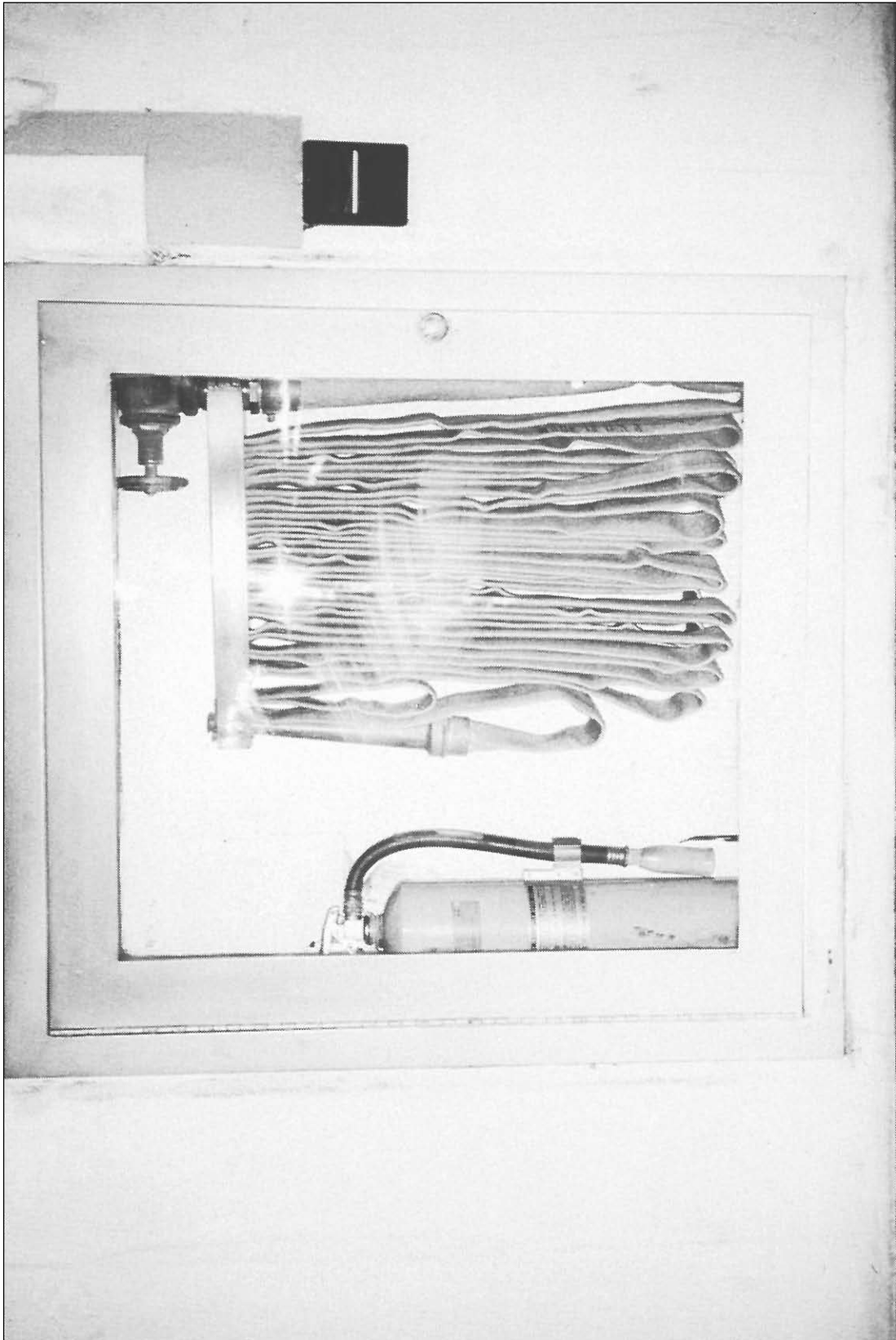
8. Typical 1 - 1/2-inch hose outlet, located at each stairwell entrance on each floor.
