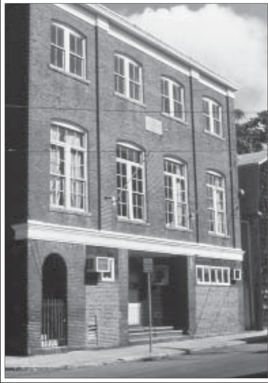
Exterior of St. Joseph Hall, 1993, before renovations.
