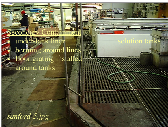
Photo: Shop Floor Showing 2° Containment Taken By: Greg V. Arthur Date: 04/04/06
