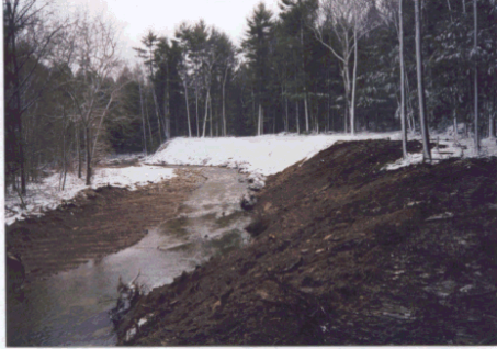
Upstream Site 1 – After completion of the project – March 1999
