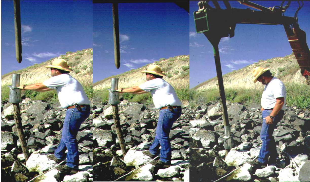
Planting a willow pole into rock riprap. In photo 1, the stinger has already punched a hole into the rock. In photo 2, the cap is placed on the pole and the stinger is guided into the hole in the top of the cap. In photo 3, the stinger pushes the pole into the pre-punched hole. The cutting will have about 1 foot sticking out of the ground when done.
