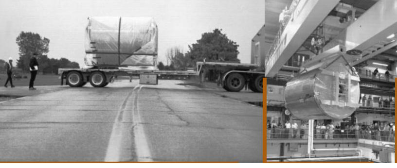
The truck trip took about half an hour (left), with the COT mounted on the same stand used for assembly in IB4. Project co-leader Aseet Mukherjee explained that the wheeled support would allow the "can" to roll in accommodating any flexing by the truck bed. The COT was then lifted by crane (right) into the CDF Assembly Hall.
