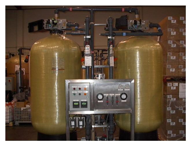
Figure A-5. Nambe Pueblo, NM Treatment System (Photograph Taken before Shipment)
