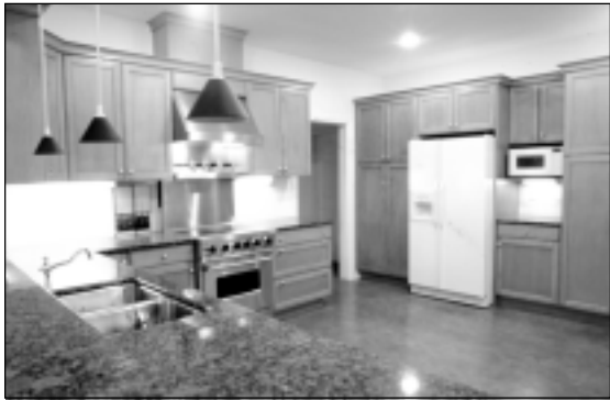
Figure 39. These attractive fluorescent lighting fixtures use one-quarter the electricity of incandescent bulbs and do not emit nearly as much heat.
