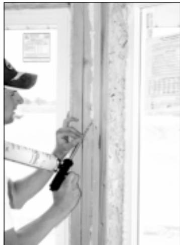
Figure 49. Air sealing around window openings.
