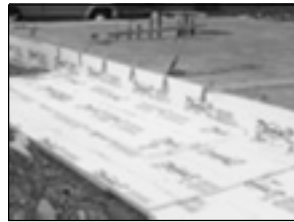
Figure 33. Frost-protected shallow foundation.
