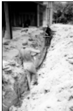
Figure 41. Workers making the loop connection to the house.
