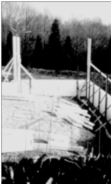
Figure 21. Insulating Concrete Form foundation under construction.
