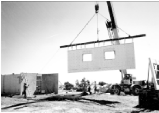
Figure 25. A concrete panel that was poured in a factory off site is lifted into place by crane.
