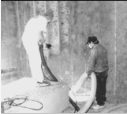
Figure 30. Workers spray cellulose insulation into a wall cavity.
