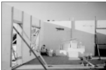
Figure 22. Insulating Concrete Form walls under construction.
