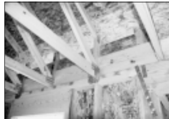
Figure 27. Raised-heel roof truss.
