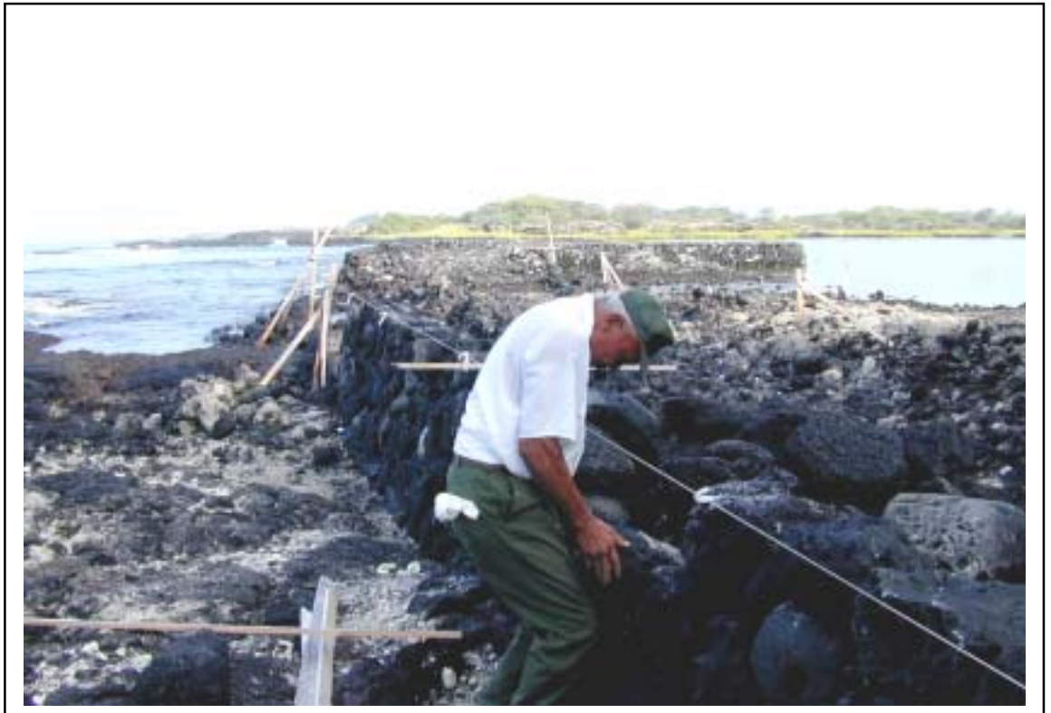
Peter Keka setting stone in the "Pā loko" (Kuapā) wall of Kaloko Fishpond (KPA Photo No. 1301)
