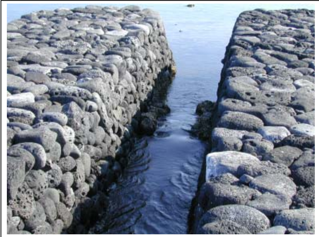
Restored Mākāhā (southern section) on Kaloko Fishpond Wall (KPA Photo No. 776)
