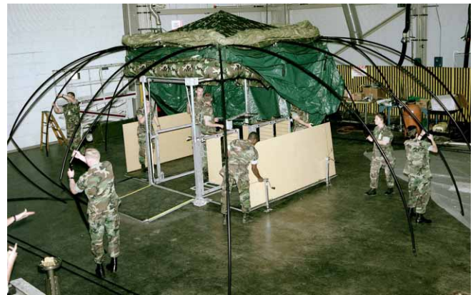
ASSTC can be deployed and operational in 30 minutes.
