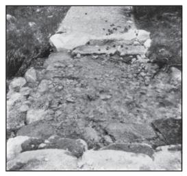
Figure 28—Wide cross drain and causeway.
