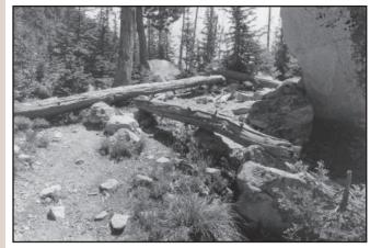
Figure 73—Abandoned trails need to be blocked off effectively, and with sensitivity.
