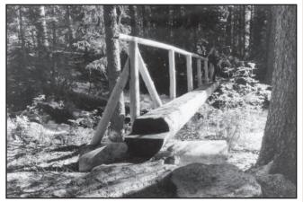
Figure 55—Log footbridge. The sill can be notched to accommodate the logs, not vice-versa.
