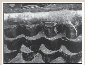
Figure 39—"Flower pot" retaining wall of geocells.
