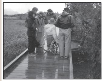
Figure 25—This boardwalk relies on pilings for support. Helical earth anchors can also support the structure.
