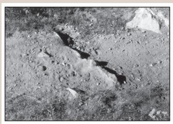
Figure 21—Waterbars need to be constructed at a 45 to  $60^{\circ}$  angle to the trail. Water should run off the trail before hitting the waterbar.
