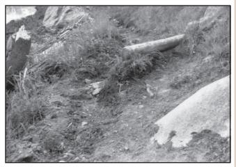
Figure 4—Too much water and sediment washed this waterbar out. Keep the water moving until you get the suspended soil where you want it. This sounds simple, but most failed water diversion structures are ones clogged with deposited soil.
