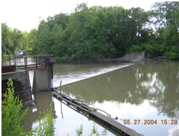
Lake Vermilion Dam and Spillway
