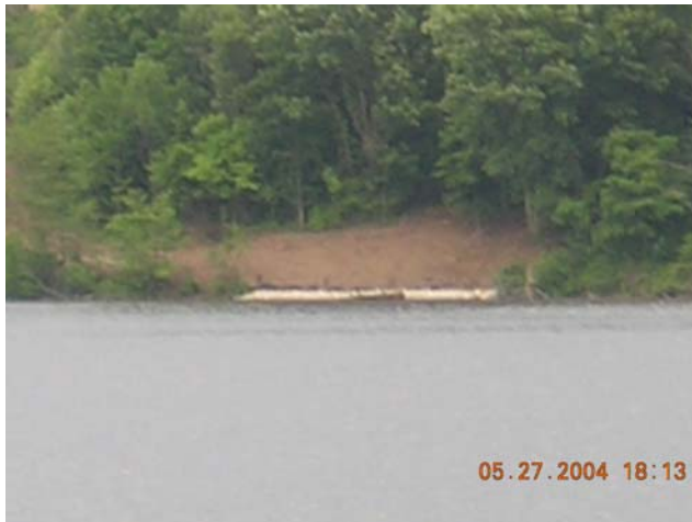
Lake Vermilion Bank Erosion
