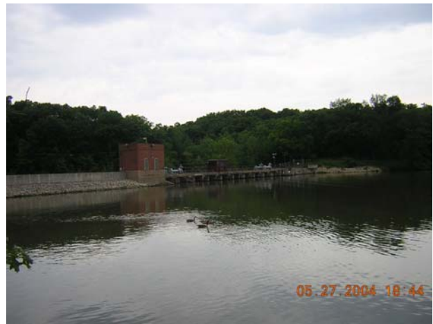
Water Plant Intake
