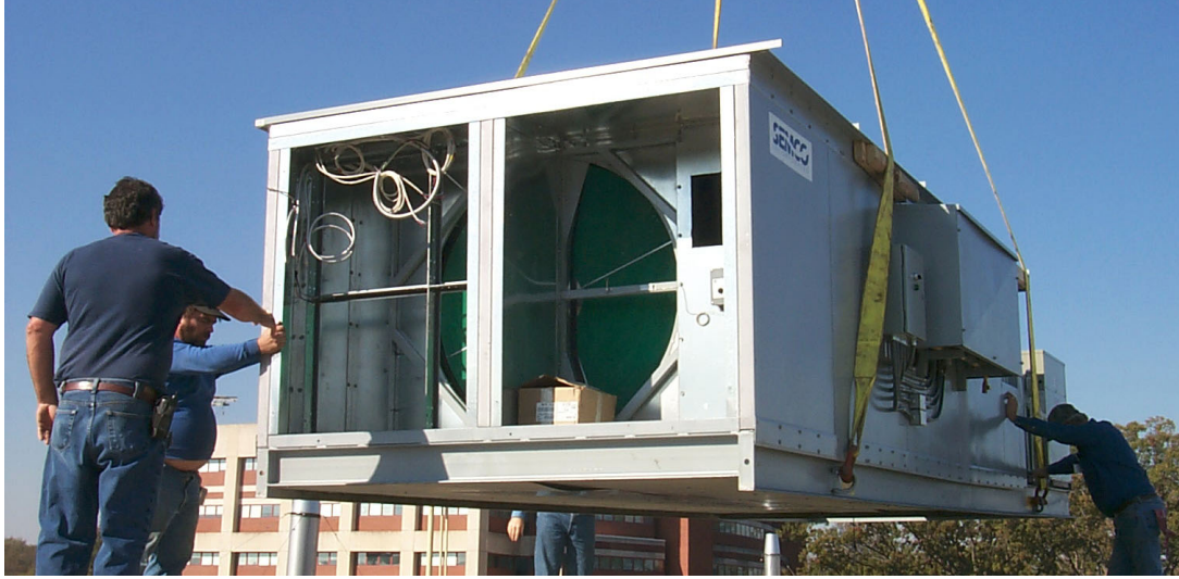
Fig. 1. SEMCO active desiccant system being installed on the Baker Building rooftop.
